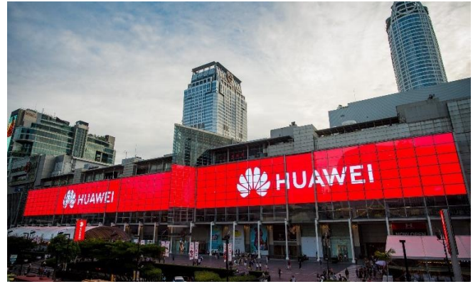
CentralWorld (ongoing renovation)
