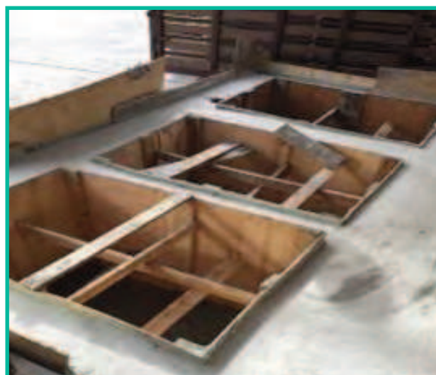
Settling basin at the boiler room
