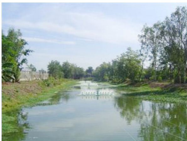
Aerating turbine system adding oxygen content in water before released to outside
