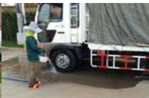
Cleaning up tires of vehicles prior to leaving a construction site to control and reduce dust emission from construction to offsite
