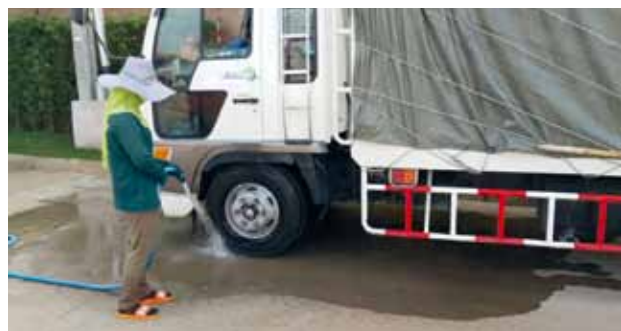
clean tires before leaving construction site to control dust spreading
