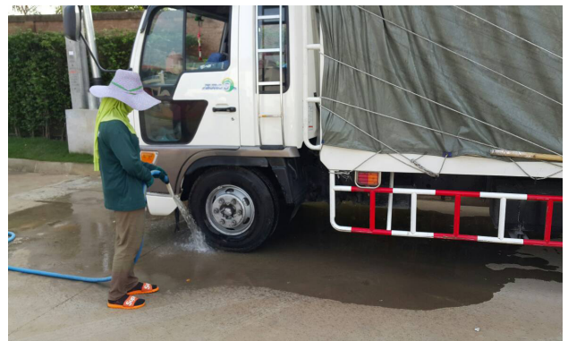
clean tires before leaving construction site to control dust spreading
