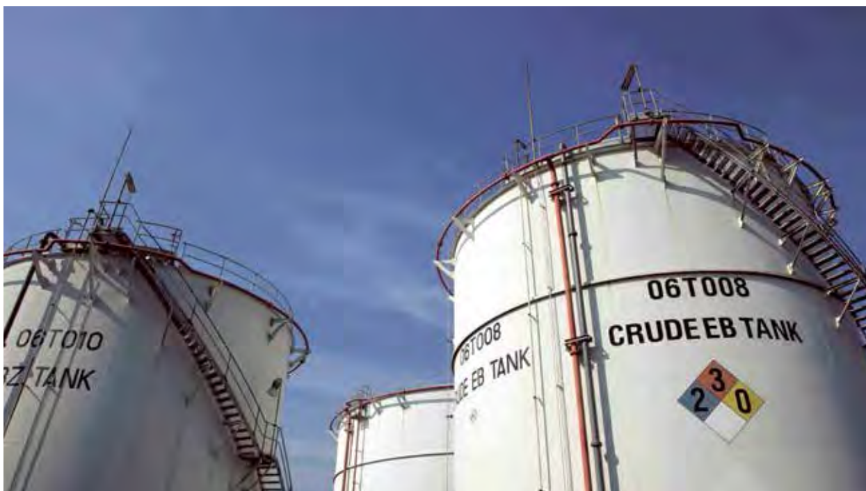
Raw material storage tanks for Ethylbenzene production unit
