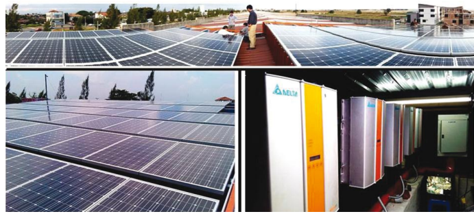
32kW Solar rooftop installed with Solivia 5.0 Solar Inverter on Commercial Shop Roof in Melaka, Malaysia
