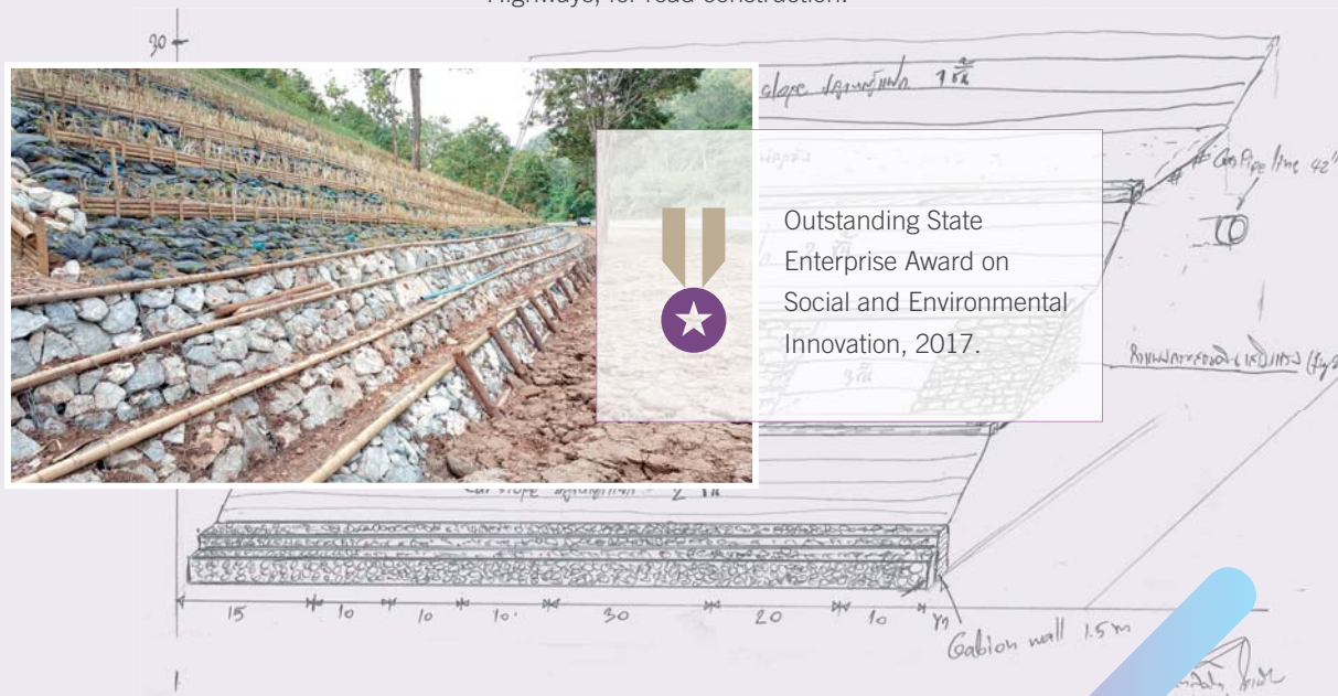
Vetiver grass implant in bamboo tubes.
