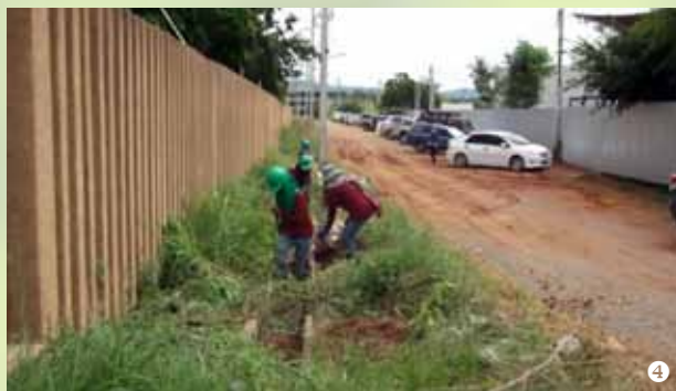
Sample 3 - Drain Clearing and Cleaning Around the Construction Project for Better Environment and Better Water Flow
