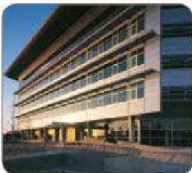
Grade SUS445M2, low-reflectivity matt finish, ASSDA, Australia
