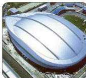
Grade SUS445J2, Kitakyushu Mediadome (Fukuoka Pref.)1998, Japan
