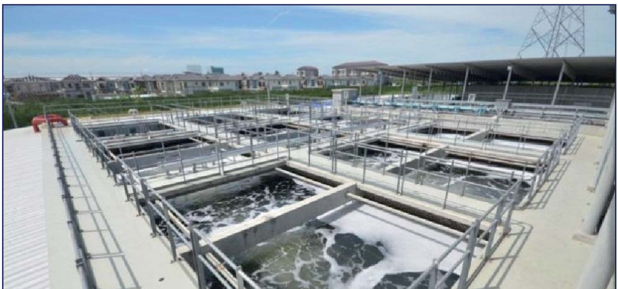
Waste Water Treatment Facilities in TOG Plant (Bio Fix Film)
