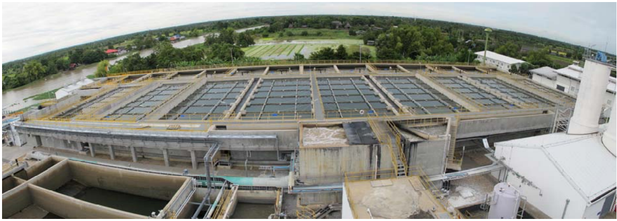
Bang Len Water Treatment Plant, production capacity of 440,000 m 3 /day
