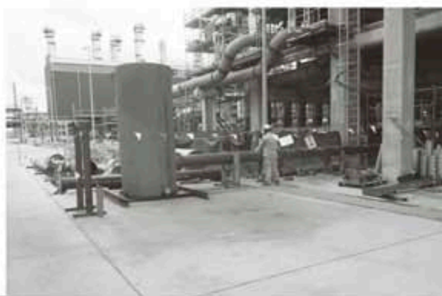
Fitting a silencer during flushing activity
