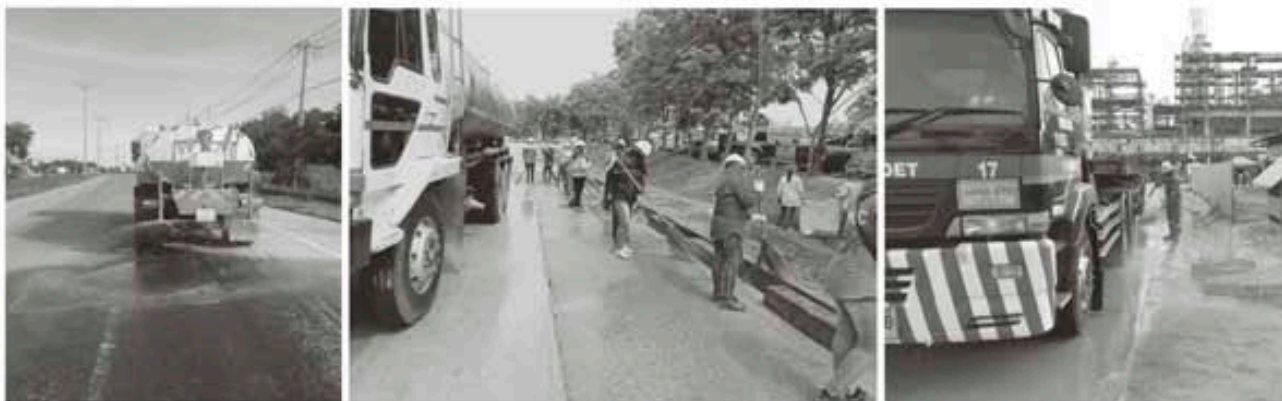
TTCL provided water spray on transportation route within the project and surrounding areas included cleaning vehicle wheels before departure from project site
