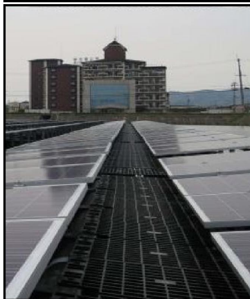
Image of a solar floating power plant project at Sirindhorn dam with a size of 256kw
