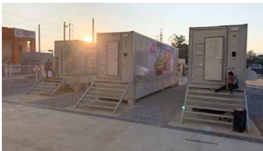
Battery Energy Storage system, size 3MW/2.2 MWh, Microgrid at Mae Sariang District, Mae Hong Son Province
