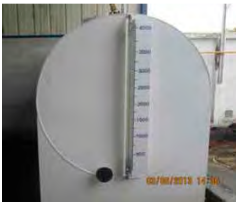
3. Filter crubed oil storage tank
