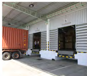
Overhead Doors With Hydraulic Dock Levelers
