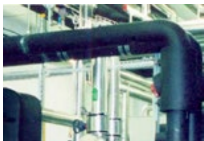
Hot water piping inside the building
