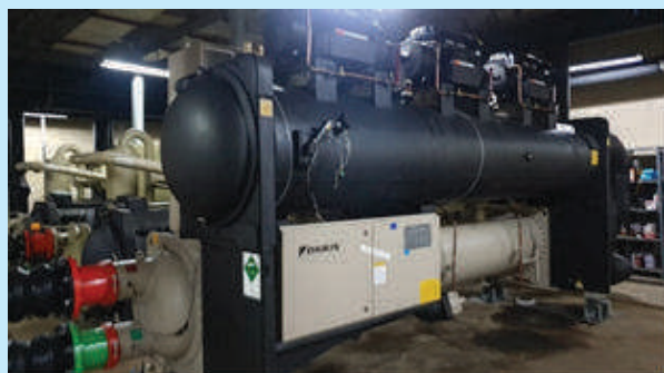
Picture 1 Change of water cooling machine to magnetic bearing cooling machine
