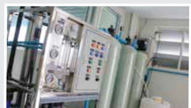
Softener, Reverse Osmosis and Ultraviolet
