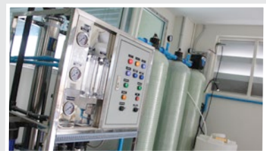
Softener, Reverse Osmosis and Ultraviolet
