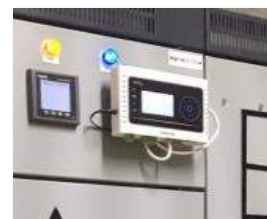
4) switchboard controller and data locker
