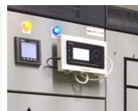
4) switchboard controller and data locker
