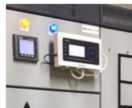
4) switchboard controller and data locker
