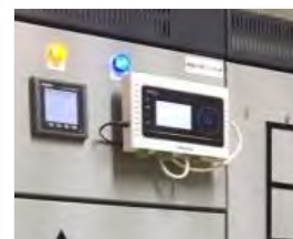
4) switchboard controller and data locker
