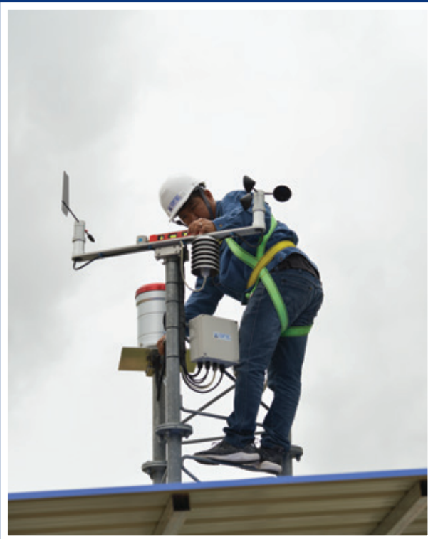
Weather Station Installation
