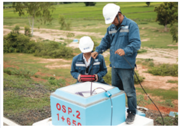
Open and Standpipe Piezometer Installation
