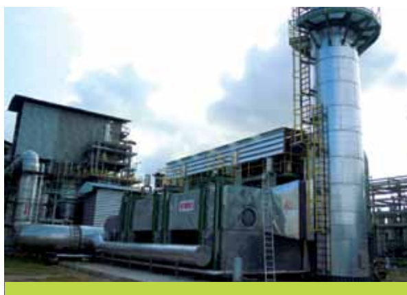
Installed the second deodorizing unit to raise operation reliability and lower environmental impacts
