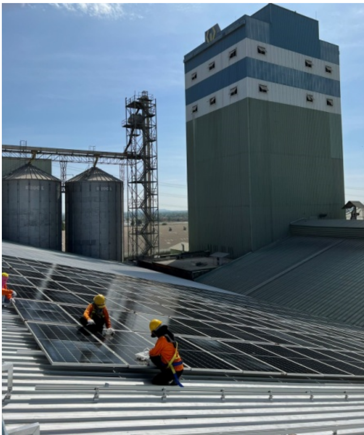
Solar panel installation process
