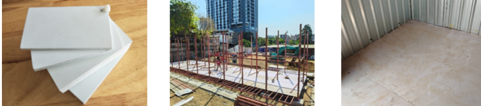
Worker accommodation using new Plastwood sheets ( Reuse 3 Times)
