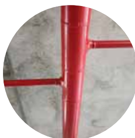
Joint fire extinguishing system pipes
