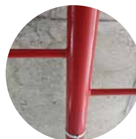
Jointless fire extinguishing system pipes
