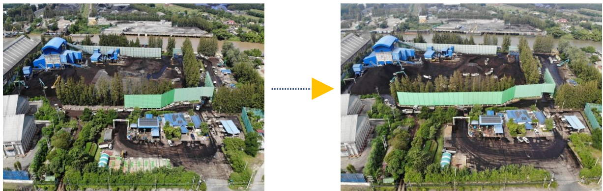
Pictures show the progress of a permanent wind break construction at the Coal Distribution Center, Phra Nakhon Si Ayutthaya Province
