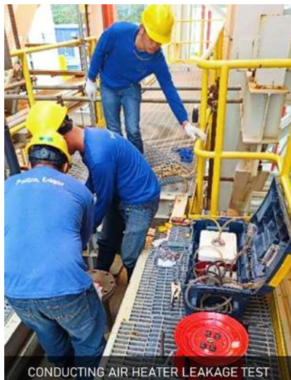
CONDUCTING AIR HEATER LEAKAGE TEST
