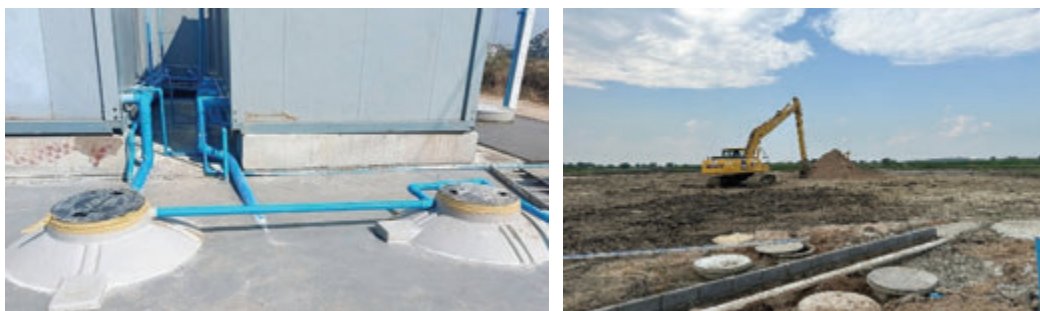
Image: Installation of wastewater treatment tanks or concrete pond systems for wastewater treatment
