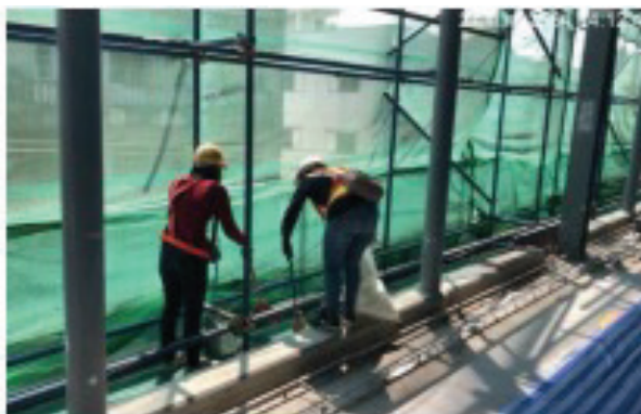
Image: Preparation of mesh to support materials from high areas
