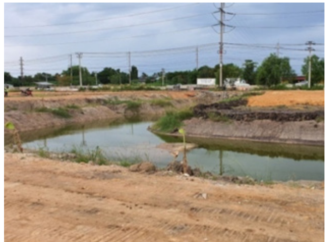
Image: Drainage way and sedimentation tank
