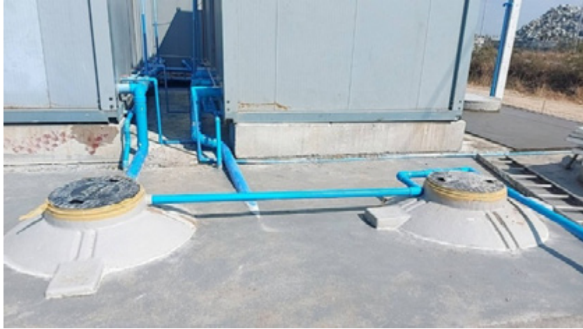
Image: Installation of wastewater treatment tanks or concrete pond systems for wastewater treatment
