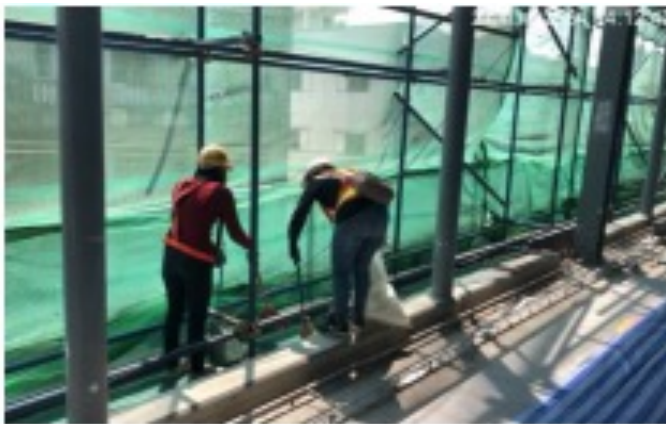
Image: Installation of safety net to catch construction materials from high-level work
