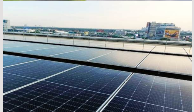
The Installations of Solar Roof at FYI Center with the Capacity of 300KW
