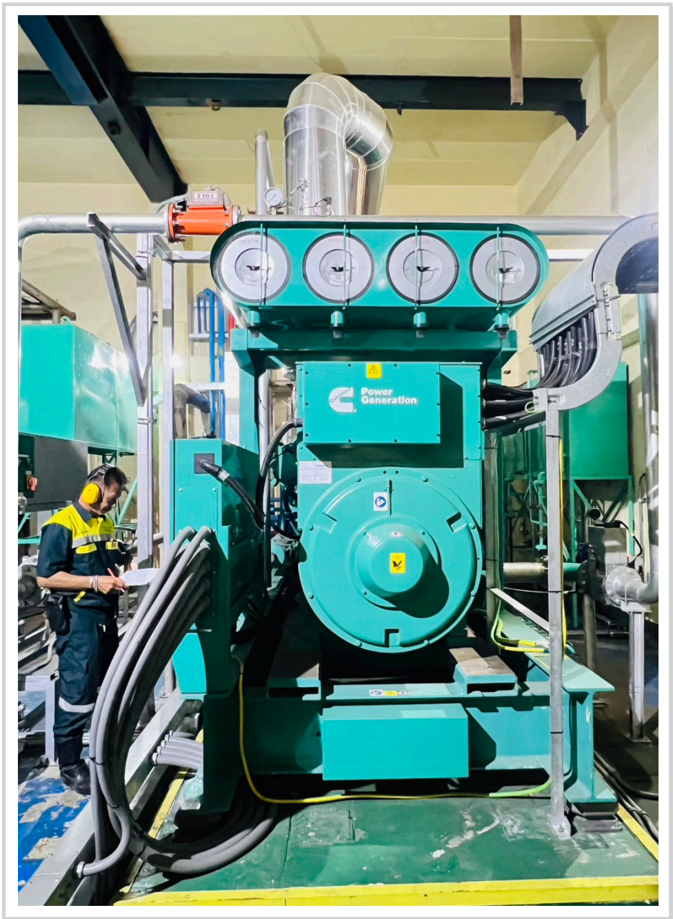
Topi Replacement Gas Engine
