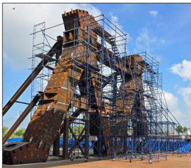
Pre-Assembly Project : Tokiwabashi Diagrid
