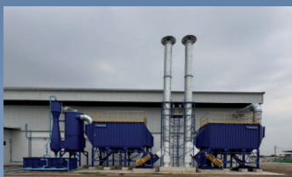
Installed a solvent odor treatment system at the CF-4 concrete tile cover and CT-6 concrete tile production line, which is a new production line.
