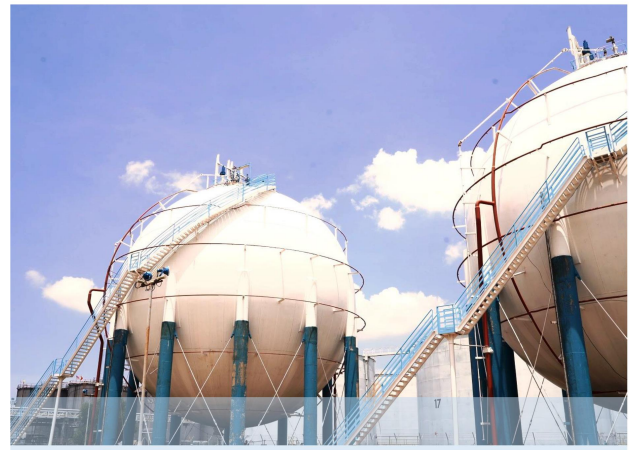
Bulk LPG storage tank
