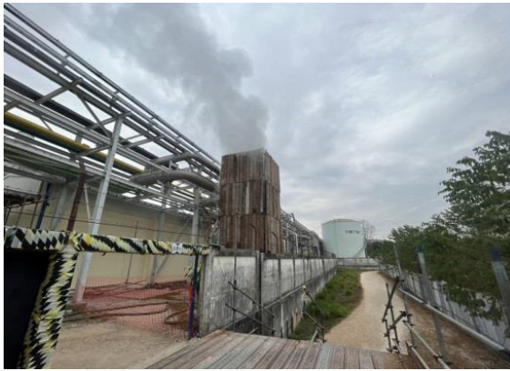
Installed a silencer in construction site
