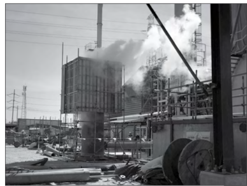
Fitting a silencer in construction site
