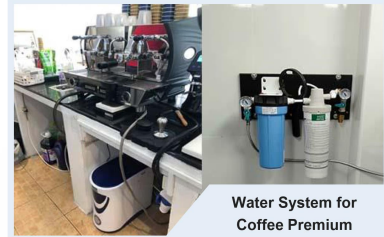
RO System (Pre Treatment Raw Water)
