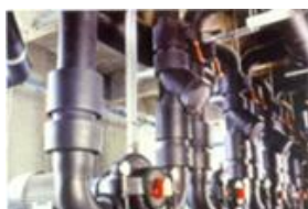
Chilled water piping
