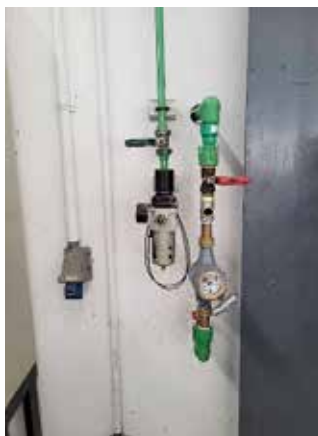
Here is an image of the water meter installation at the workshop, showing how the water usage is measured separately for workshop activities.
