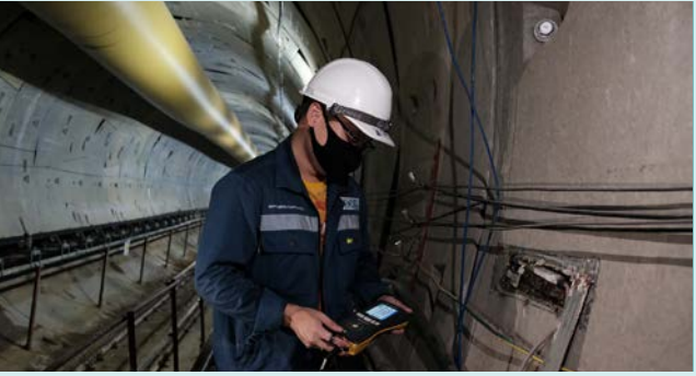
Total Pressure Cell Monitoring in Tunnel
