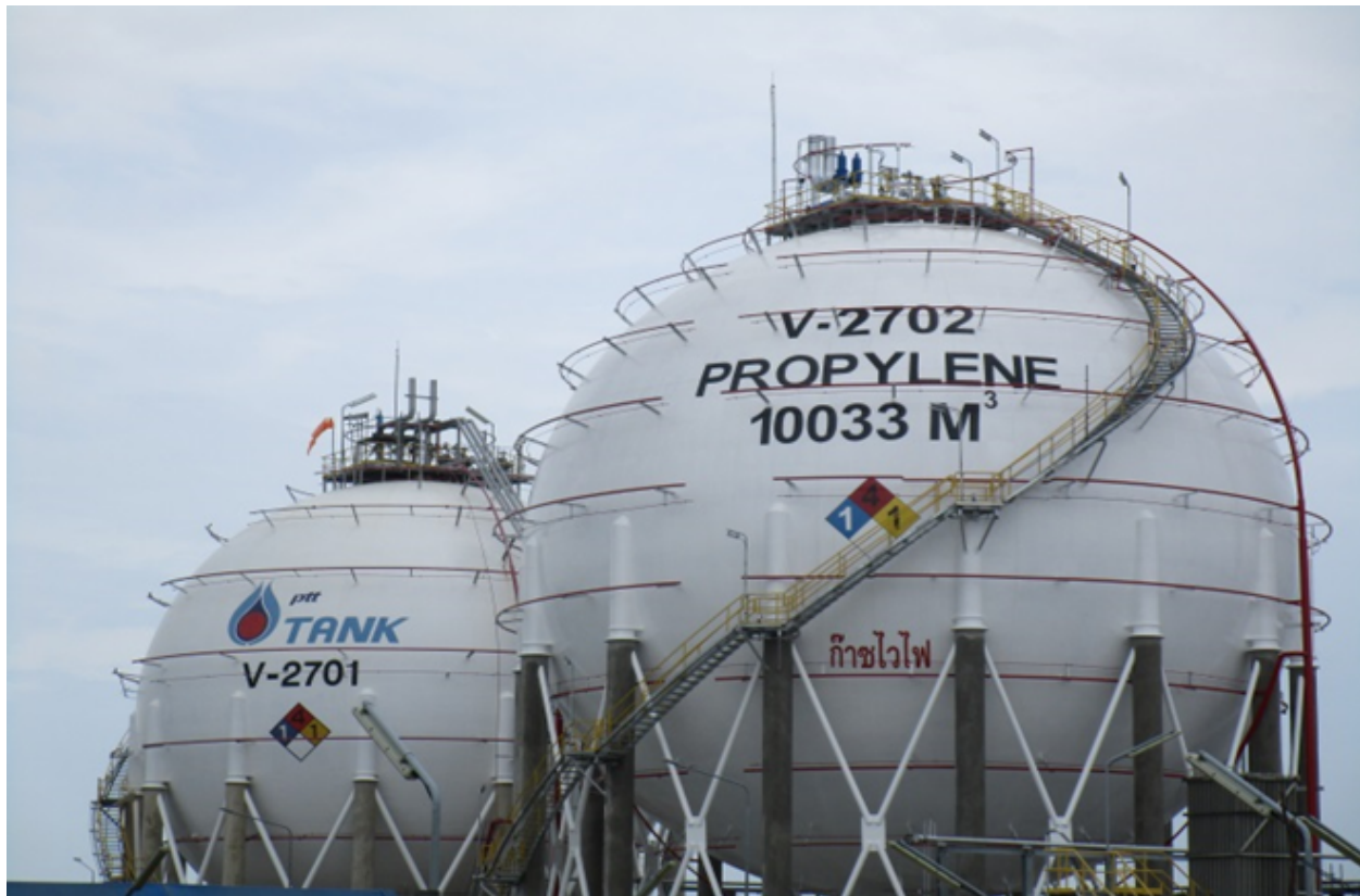
PTT Tank Terminal Propylene Spherical Tank: Propylene Storage 4,000 tons
