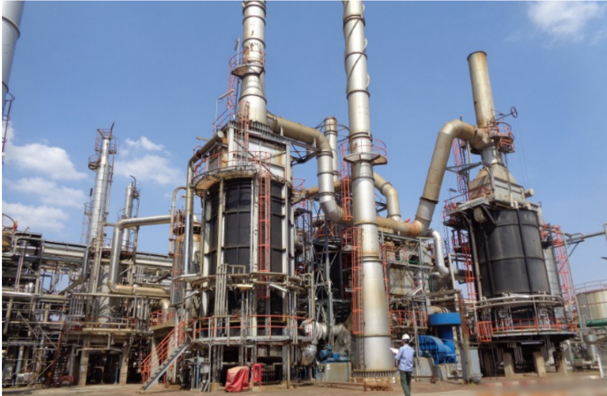
Bangchak Refinery Upgrade Project for Environmental Excellence or 3E Phase 2: Installation of New Continuous Catalyst Regeneration (CCR) and Hydrocracker Unit (HCU)
