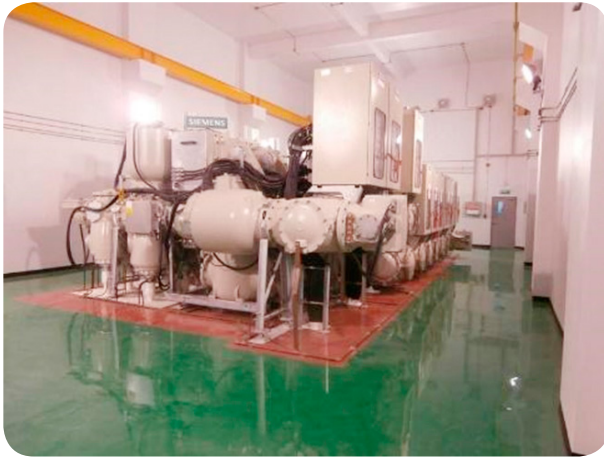
GAS-INSULATED SUBSTATION (GIS)
