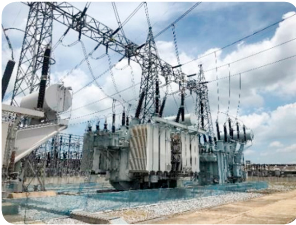
AIR-INSULATED SUBSTATION (AIS)
