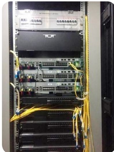
THE INSTALLATION OF MSAN SYSTEM AND EQUIPMENT
