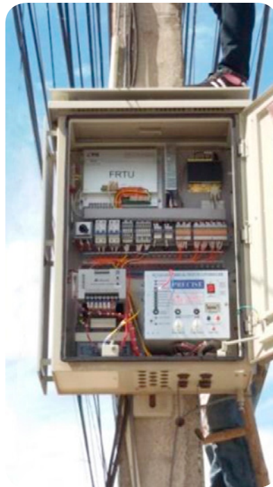
FRTU SYSTEM INSTALLATION
