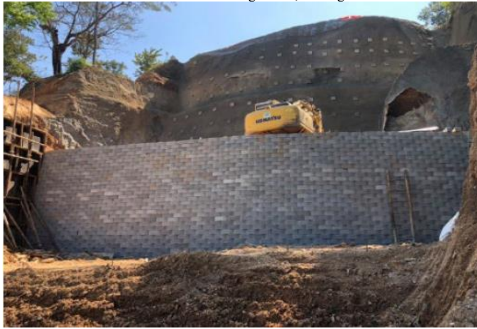
Slope Protection Work of Highway No.1322 Control Part 0100 Part Mea Ja– Rin Luang Part 2, Chiang Mai
