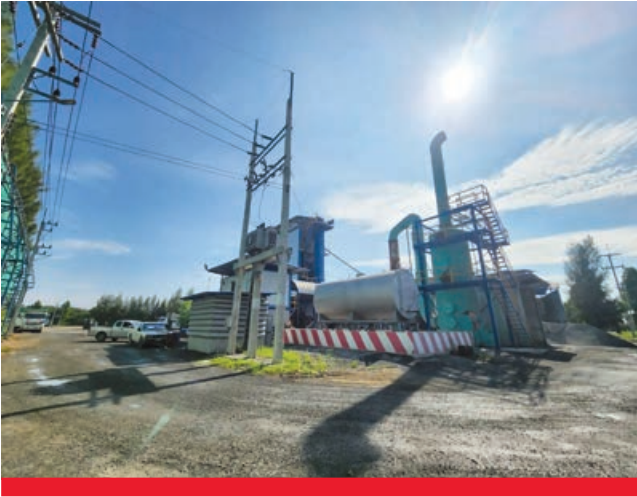
Image: wet Scrubber at asphaltic concrete plant
